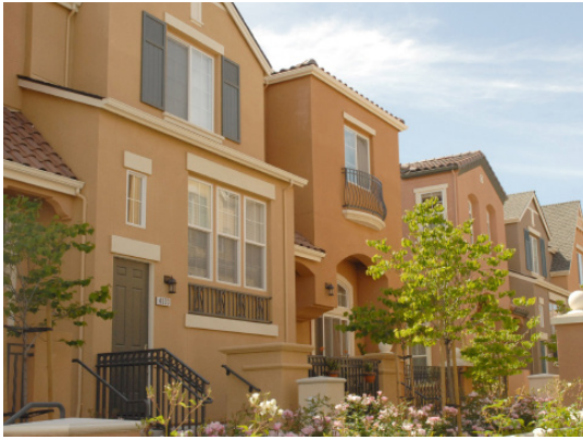
Medium density housing types, such as townhomes, will help establish a “critical mass” of residents in the new neighborhood.
