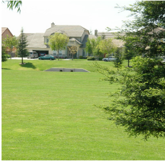
Detention basins are distributed throughout the City, capturing runoff during stormwater events. Some of these detention basins also serve as City parks.
