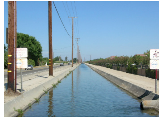
There are no natural defined streams in the Planning Area. Three open irrigation canals, TID Laterals 3, 4, and 5, pass through the Planning Area from east to west, spaced apart by two and a half miles.
